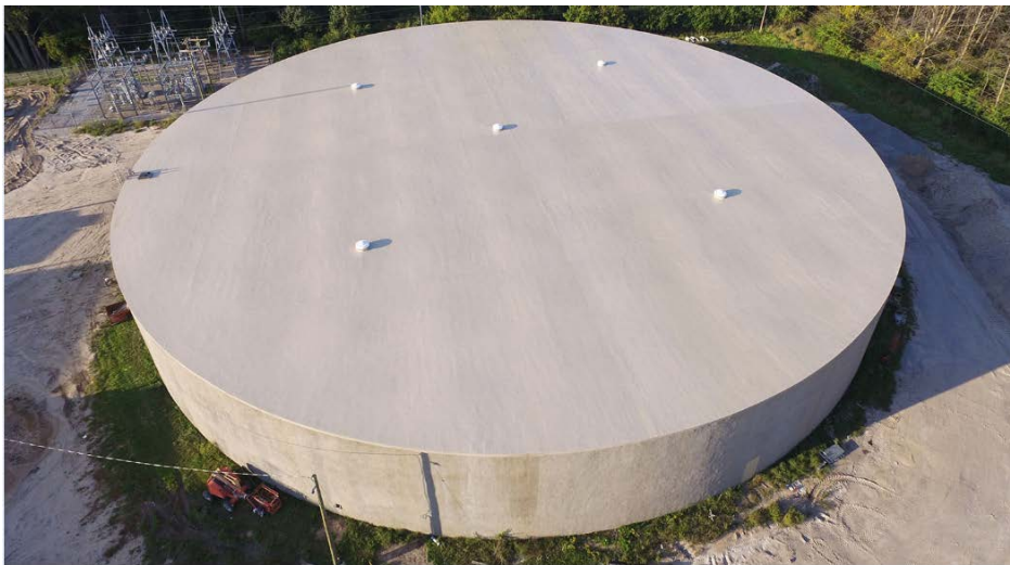
10 Million Gallon Raw Water Storage Tank
